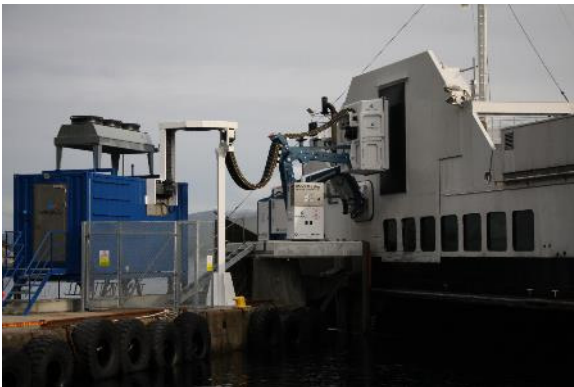
Figure 28 (Top) Pantograph, example Stemmann Technik; (middle) automatic plug-in, example Cavotec; (bottom) wireless inductive charging, example Wartsila
