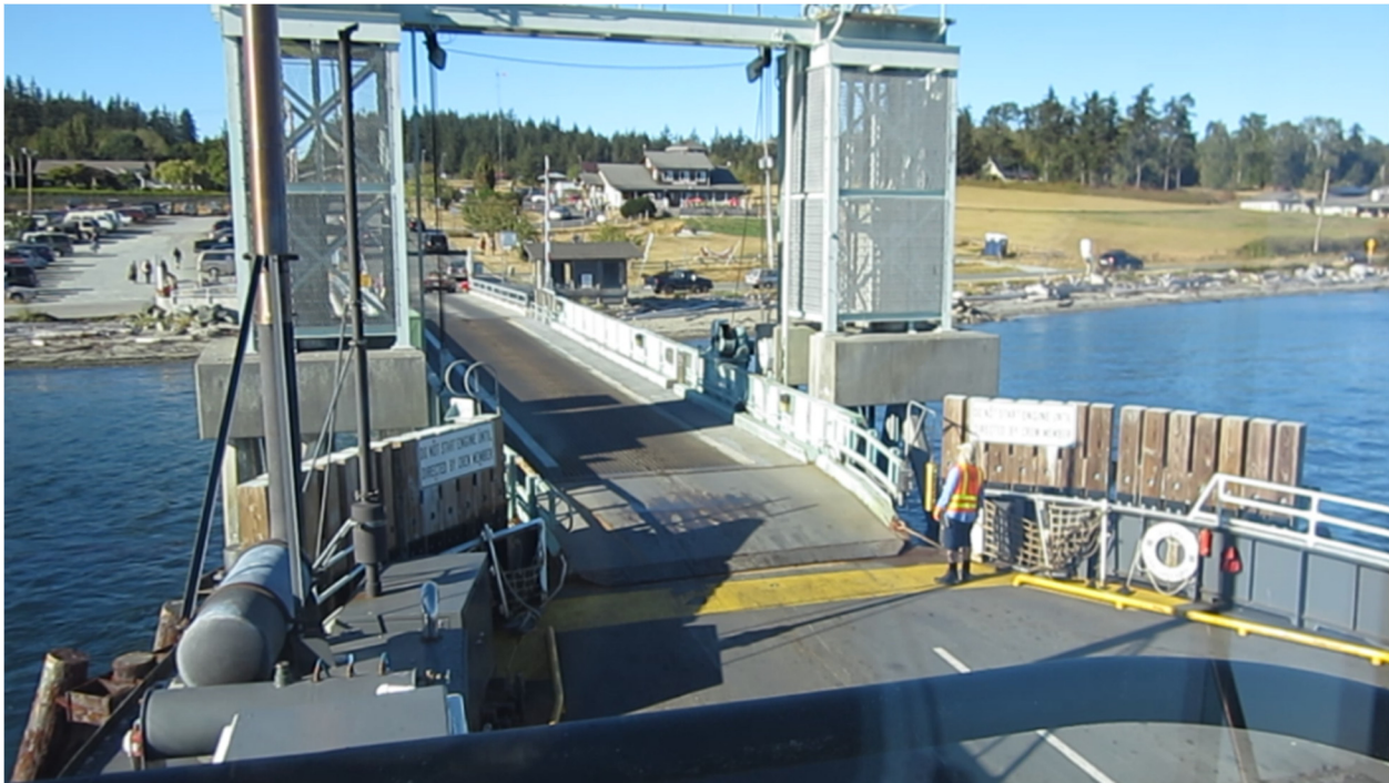
Figure 41 Guemes Island Ferry Terminal, Guemes Island
