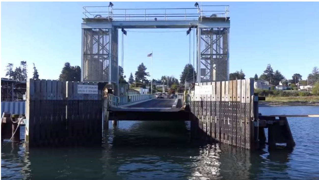
Figure 42 Guemes Island Ferry Terminal, Anacortes
